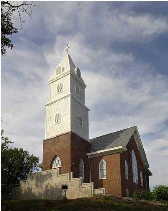
Example of a well-designed bell tower WCF
