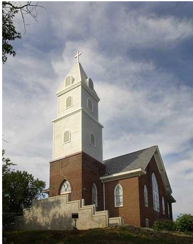
Example of a well-designed bell tower WCF
